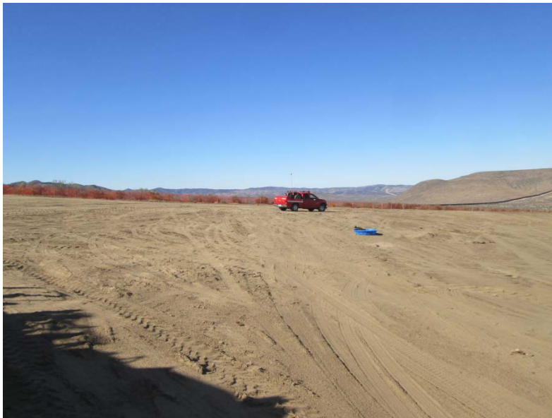
Photo 6: In accordance with MM-FF-1 and the Construction Fire Prevention/Protection Plan, SDG&E maintains ongoing fire patrols during construction activities.
