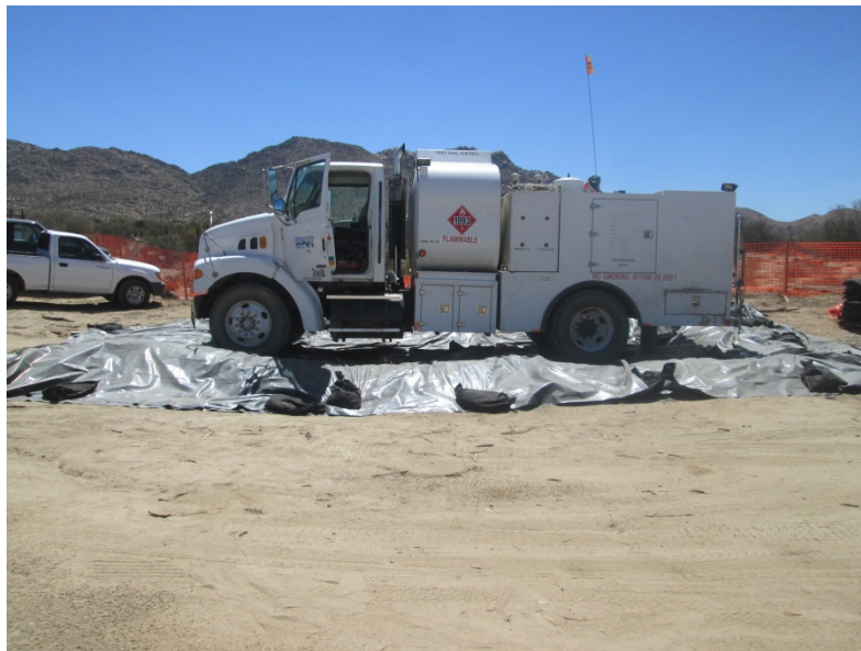
Photo 4: A secondary containment has been installed around the perimeter of a refueling truck when not in use in accordance with MM-HAZ-1A and the Hazardous Materials Management Plan.
